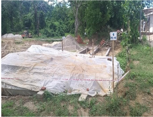
Material storage yard. Steel keeps under cover
