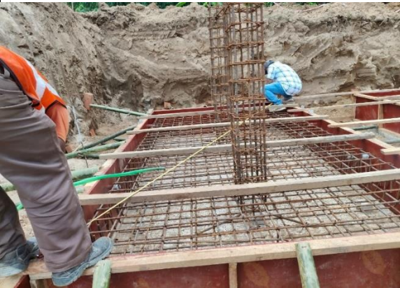
Rod Binding work under process
