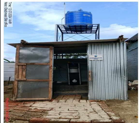
Drinking Water Facility For Labour/ Staffs
