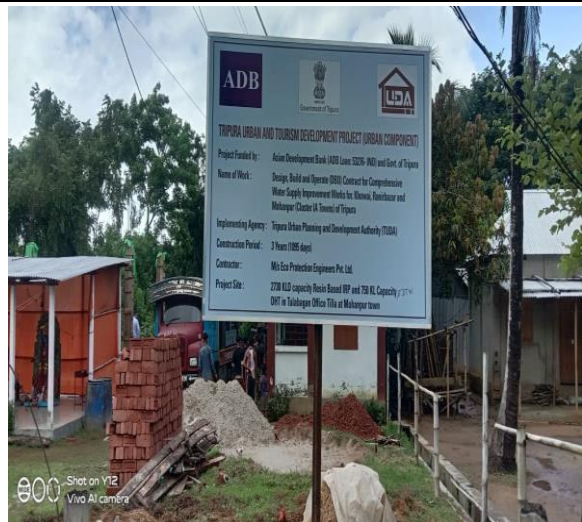
Project display board – noted at work site at Mohanpur
