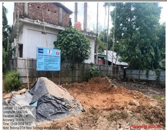
Proposed DTW location near Satmura Match Factory installation of project information board noted
