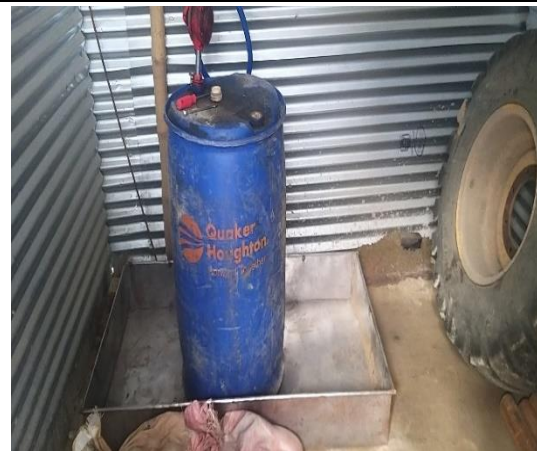
Proper storage of fuel drum. 110% containment volume metal tray noted.
