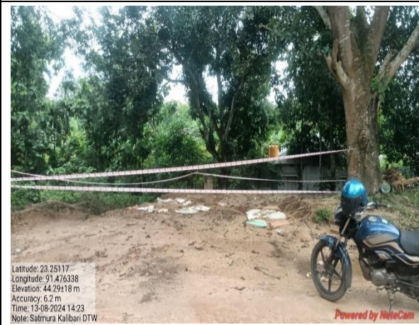
Installation of DTW near Satmura Kalibari has been Completed
