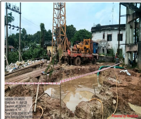
Drilling, Pipe Lowering and washing work of DTW is going on
