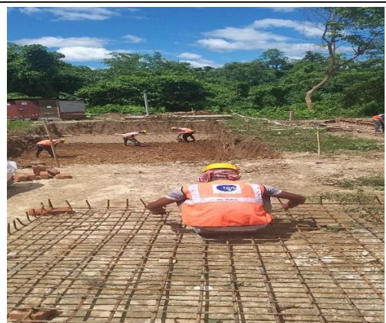
Shuttering of boundary fencing beam – under progress
