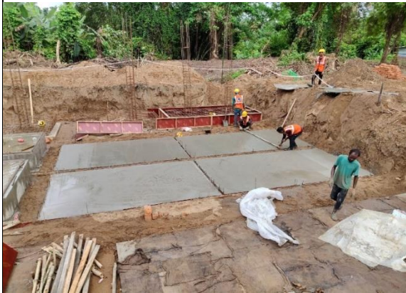
Slab Casting
