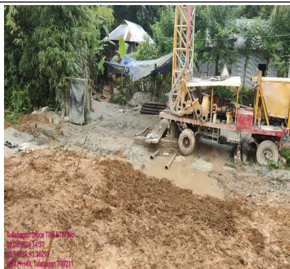
DTW Bore Wash work is going on at Mohanpur
