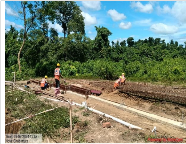
Construction of Boundary wall work - noted use of PPE kit by the workers
