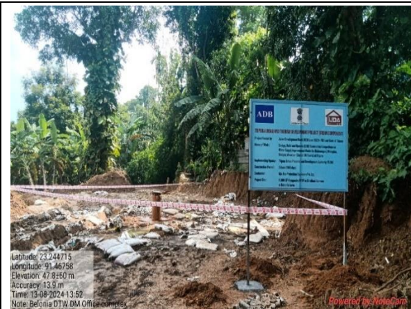
Installation of DTW back side of Narayan Smiriti Community Hall has been Completed & installation of project information board noted
