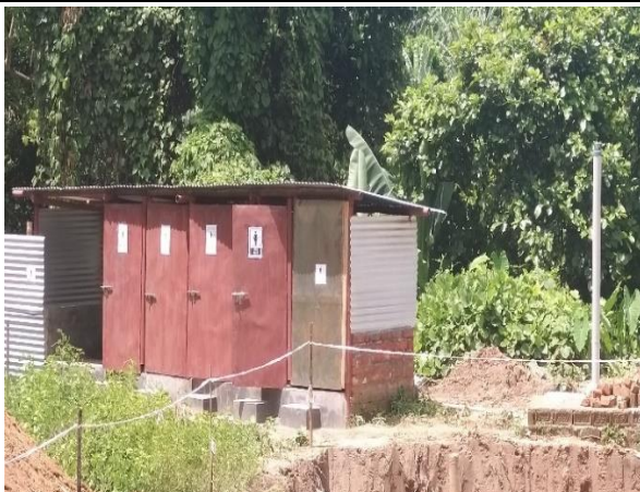
Toilet facility noted with labour camp. Separate arrangements have been made for male and female. Arrangement of water is required.
