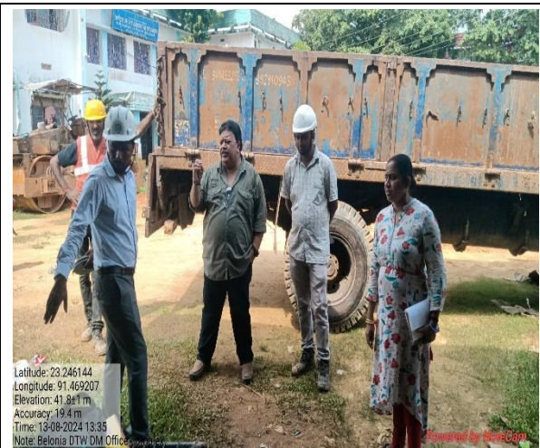
Consultation with Site Engineer and Site manager at Construction site
