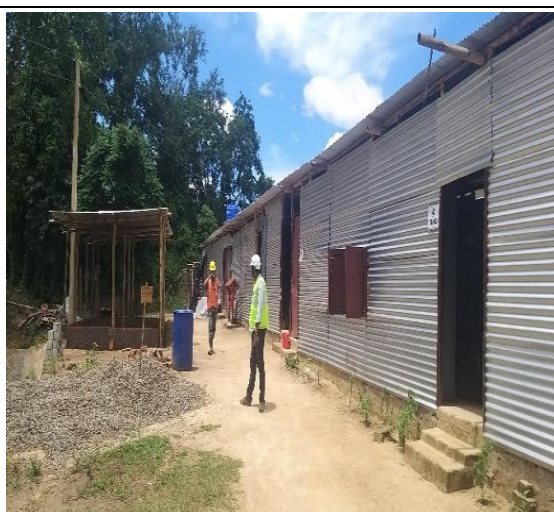
Site office, store, laboratory at Chabimura
