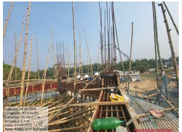
400KL OHSR Khowai 2nd Brace Beam Reinforcement and Shuttering checking
