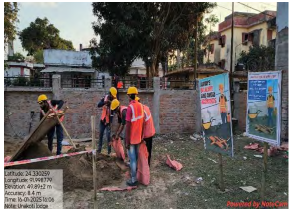
Construction work ongoing at Unakoti lodge. Signage - noted
