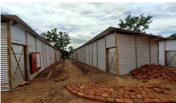
Worker's camp constructed at project site
