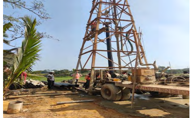
DTW ERW Pipe lowering work done in Ranirbazar
