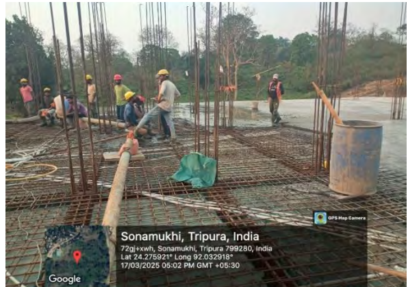
Concreting is in progress at Banquet hall lower ground floor roof slab at Sonamukhi Site
