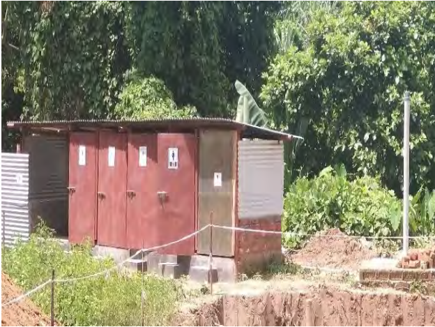
Toilet facility noted with labour camp.
