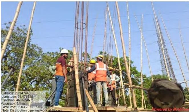
Abul kalam Community Hall @400 kl OHSR Site, Belonia Pile Cap Foundation Reinforcement Cutting & Bending Work is in Progress.
