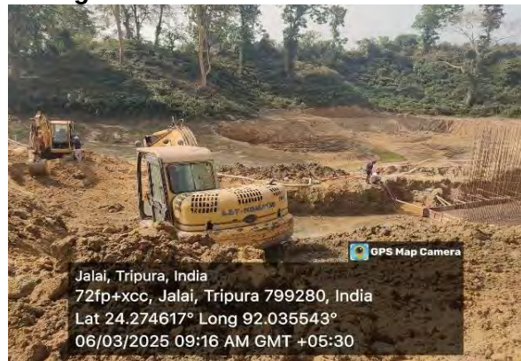
Earth excavation of retaining wall work in progress
