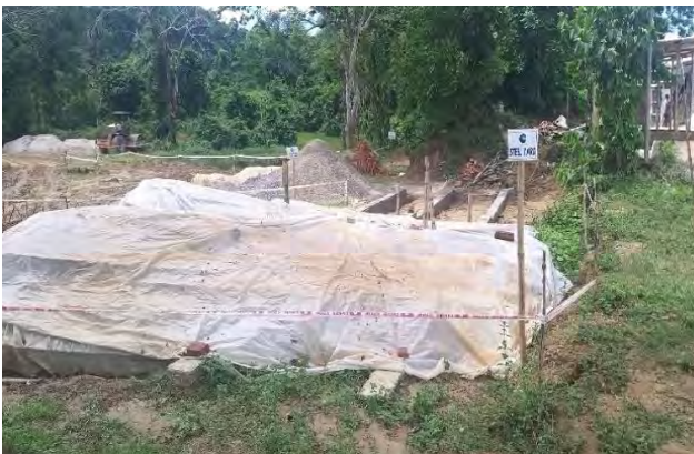
Material storage yard. Steel keeps under cover
