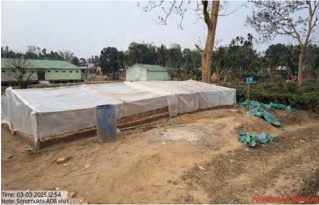
Top soil preserved and covered by terpolymer at Sonamukhi site
