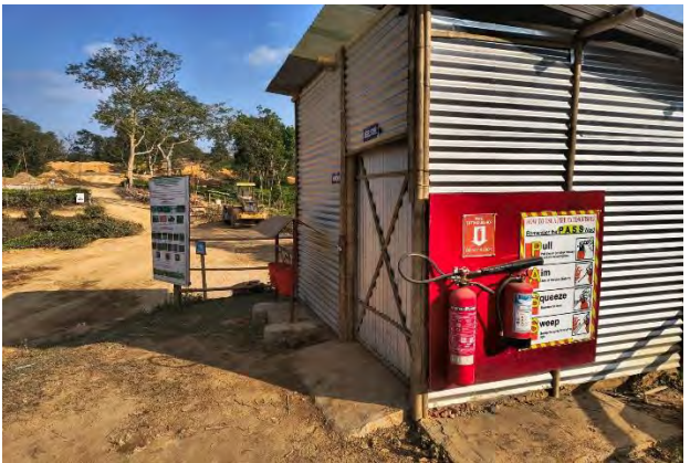
Provision of fire extinguishers at Sonamukhi site with proper signage
