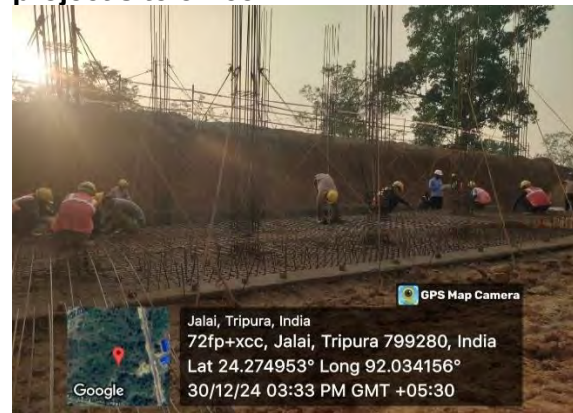
Reinforcement binding of footing grid 1 at admin building in progress
