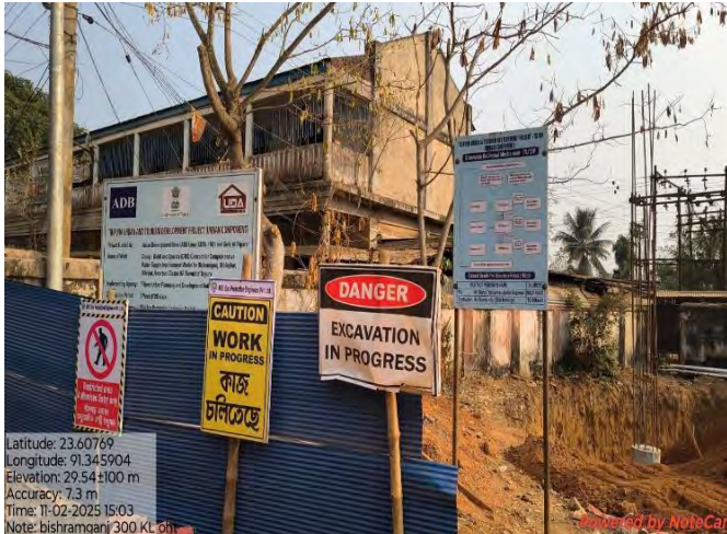
Signage is provided at cluster IIA water supply project site
