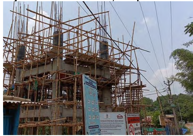
Scaffolding work at Melaghar OHSR (450kl) site
