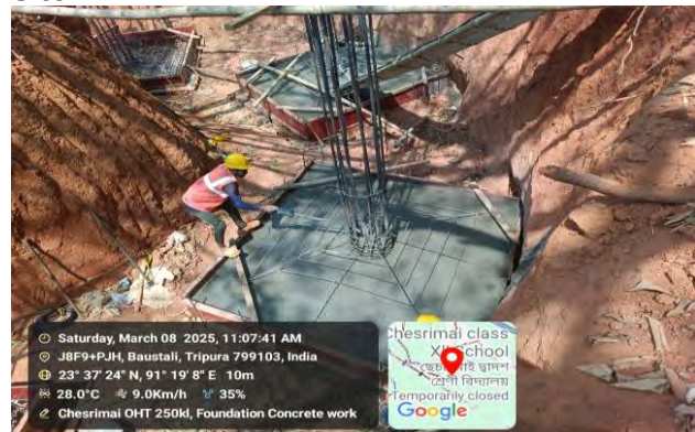
Foundation Concrete Work Is in progress at Chesrimai, Bishramganj 250kl OHSR Site.
