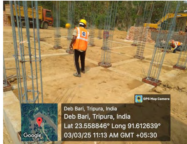
Eco Cottage 3 column starter fixing at site Chabimura
