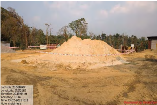
Proper demarcation of stored material at Chabimura site
