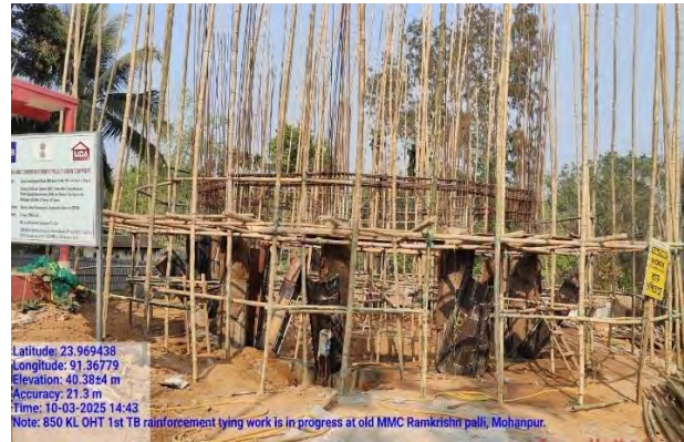
850 KL OHSR 1st TB reinforcement tying work is in progress at old MMC Ramkrishna palli, Mohanpur. Project display board is noted.
