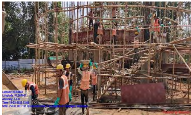
1st TB Concreting Work is Going on at 750kl OHSR Site Tulabagan Mohanpur. Use of PPEs - noted
