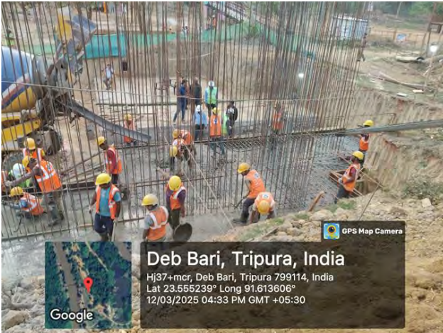
Casting is under progress at Chabimura Site. Use of PPEs by the workers – noted
