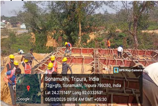
RCC casting of floor slab at suite cottage 3 started at Sonamukhi Site. Use of PPEs by workers - noted
