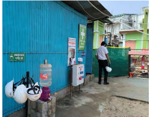
Proper labour hutment set up with provision of fire extinguishers and drinking water at Rajarshi Town Hall OHSR, Udaipur
