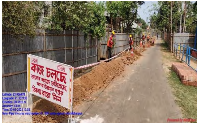
HDPE Pipe line work at area ward number-01 Mohanpur, BSF camp, opposite side- just started
