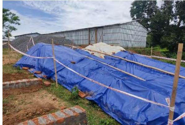
Steel storage yard. Properly covered.
