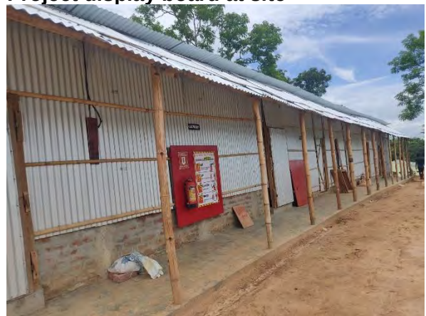
Site laboratory and worker's camp
