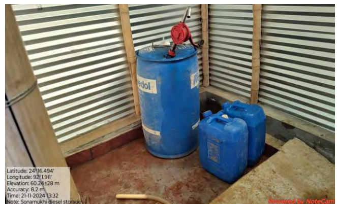
Fig. 6a, 6b: Diesel Storage room with proper diesel storage. Metal tray placed below the storage drum. Fire extinguisher available
