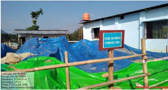
Fig. 8: Proper steel material storage area
