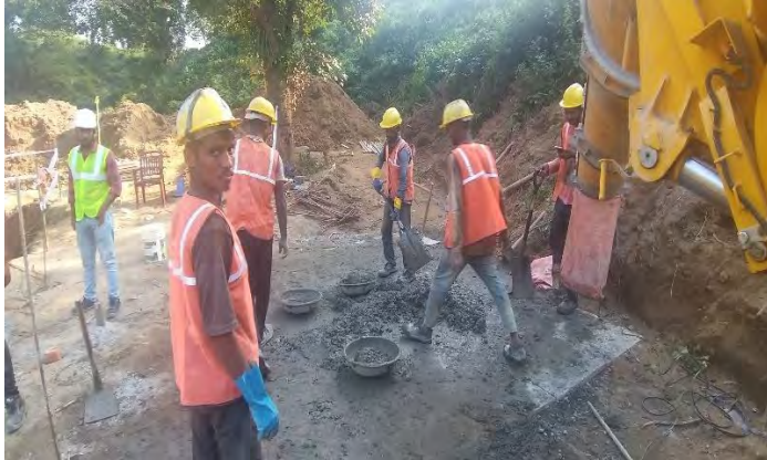
Fig. 13: Complete use of PPEs by workers during concreting work
