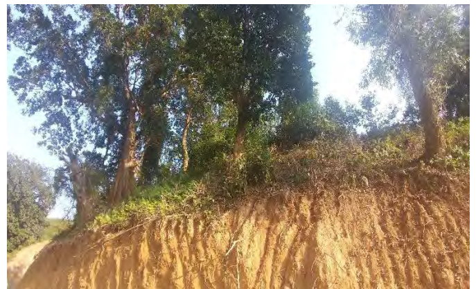
Fig. 16: Trees are saved through proper selection of road alignment
