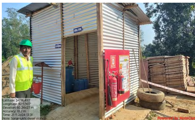
Fig. 6a, 6b: Diesel Storage room with proper diesel storage. Metal tray placed below the storage drum. Fire extinguisher available
