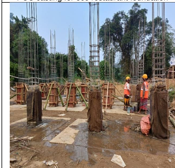
Female Worker engaged in construction work
