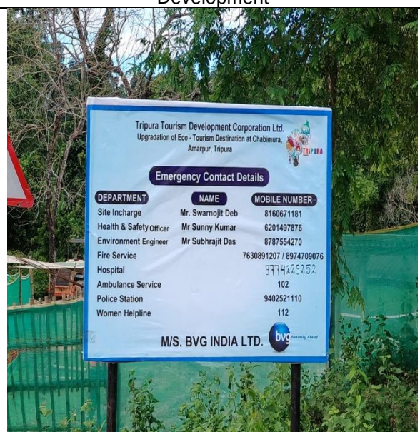
Installation of Board consisting of Emergency Contact Number
