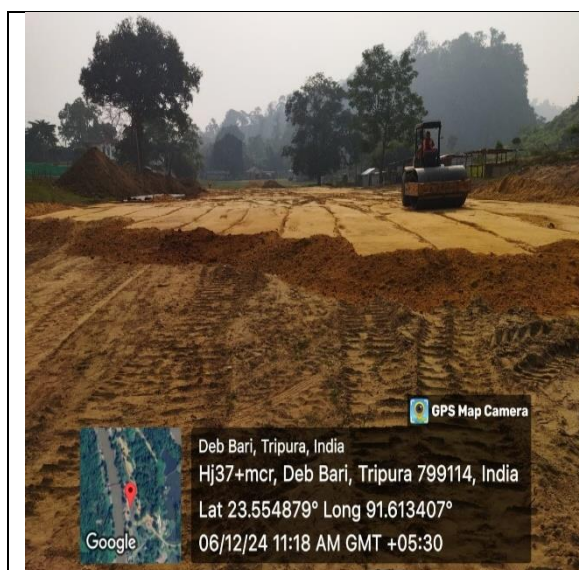
Land Levelling work is going on
