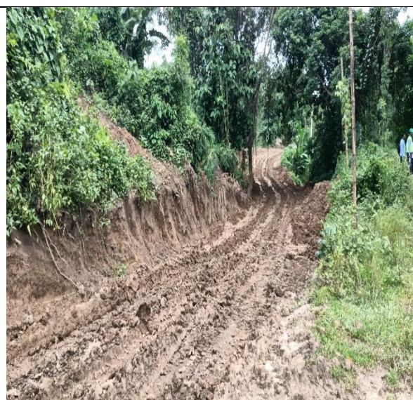
Land Levelling work is going on for Pathways Development
