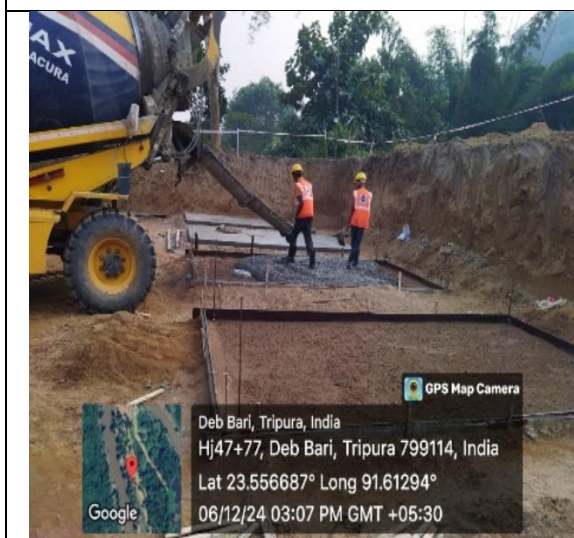
PCC casting for eco restaurant foundation
