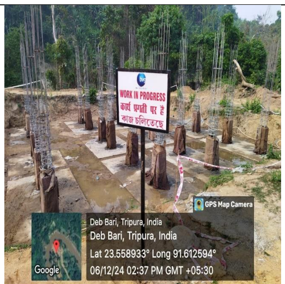
Gunny bag curing of column 1st lift at eco - cottage-4
