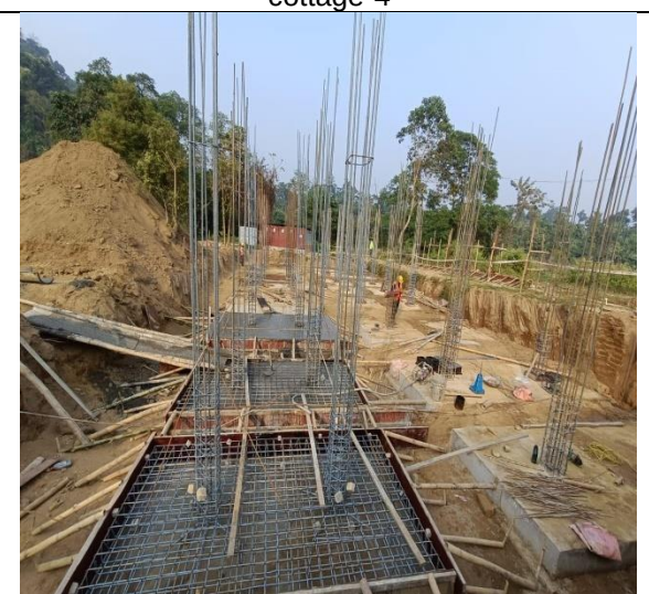
Foundation casting of staff quarter foundation
