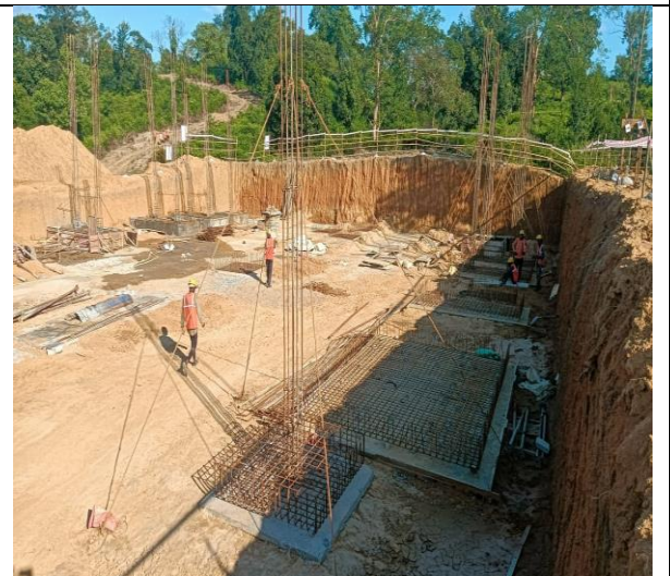
Construction work of Admin Building is in progress
