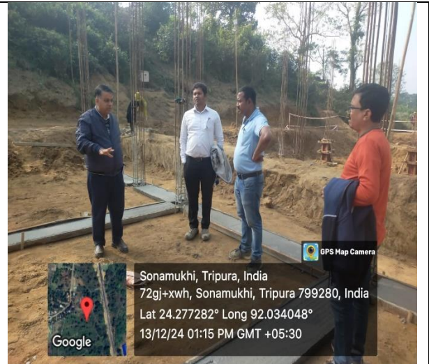
Construction work of Manager Quarter is in progress
