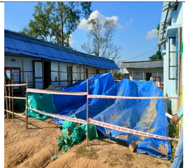
Construction Site Demarcated with Caution Tape
