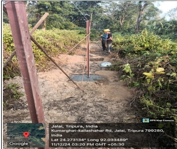
PCC and vertical angle fixing at south side Fencing work in progress
