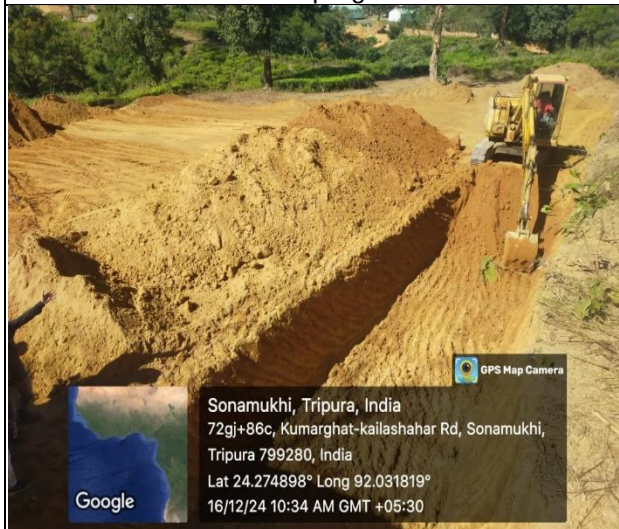
Earthwork in excavation continues at Admin building.
