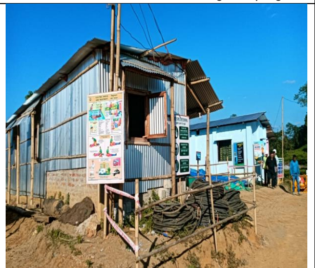
Contractors Site Office
