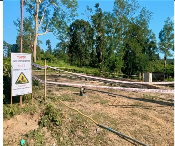
Construction Site Demarcated with Caution Tape
