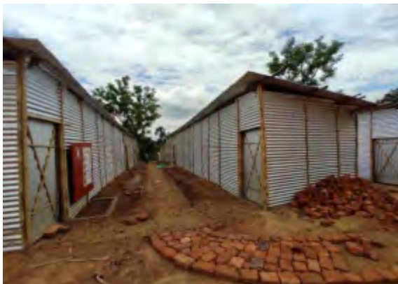
Worker's camp constructed at project site
