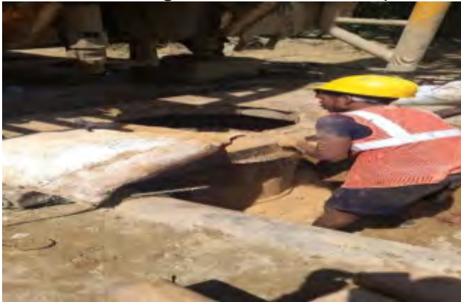
DTW work just started at Belonia – near Dr. Abul Kalam Azad community hall
