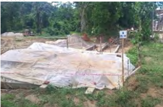
Material storage yard. Steel keeps under cover
