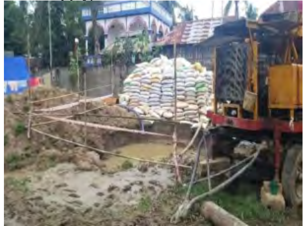
Slurry and muck collection pit at Tube well site. Caution tape placed near excavated area
