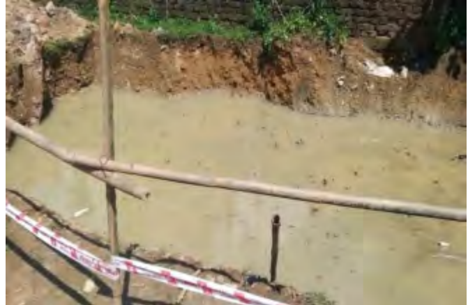
Waste water and muck stored at site, which will be discharge
