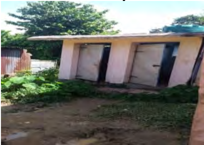
Toilet facility at DTW site - Belonia
