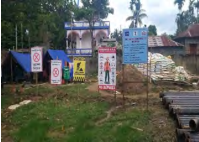
Project display board, safety signage noted at Ranirbazar DTW work site near cremation ground
