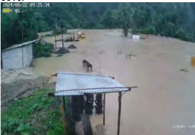
Work area flooded from Gomati river in the month of August 2024
