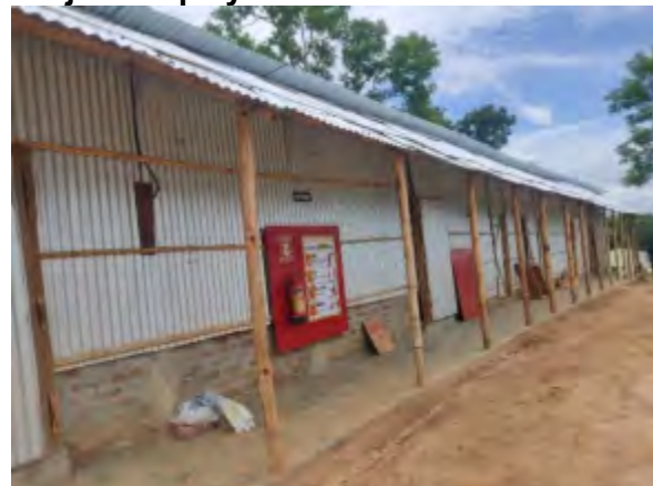
Site laboratory and staff camp
