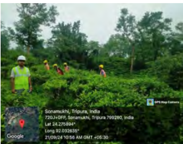
Vegetation cleaning work in progress
