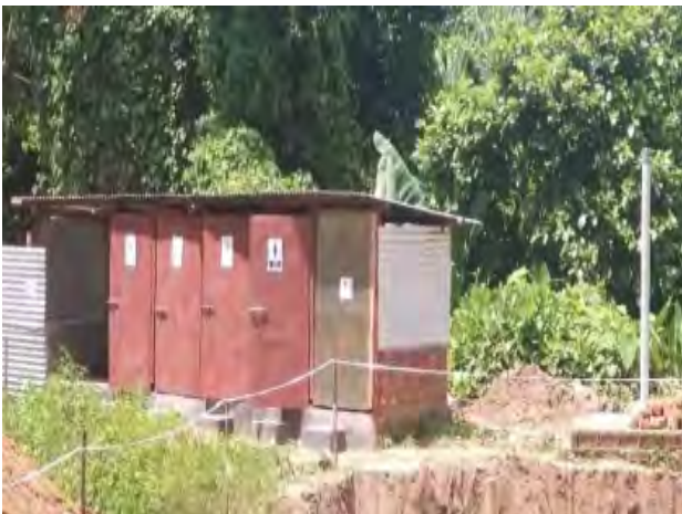
Toilet facility noted with labour camp. Arrangement of water is necessary
