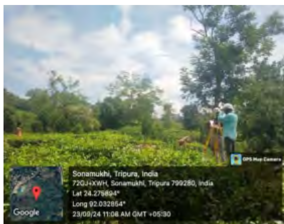
Surveying and layout marking work in progress
