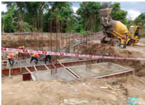
Concreting work for Eco Cottage. Use of PPEs by workers – noted
