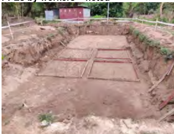
Staff quarter PCC bed preparation – under progress
