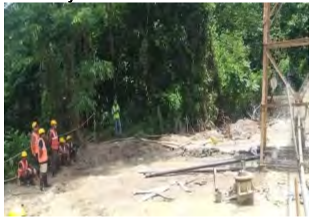
Cleaning process of tube well is under progress. Use of PPEs by the workers noted at site
