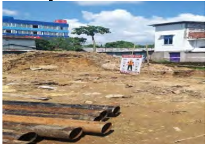
Safety signage noted at site
