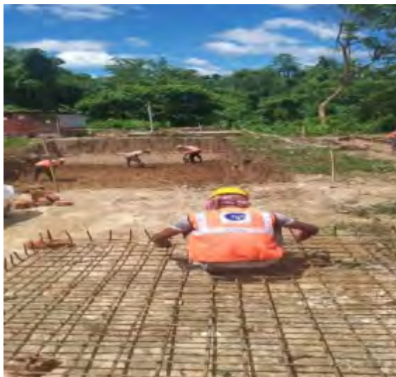
Shuttering of boundary fencing beam – under progress
