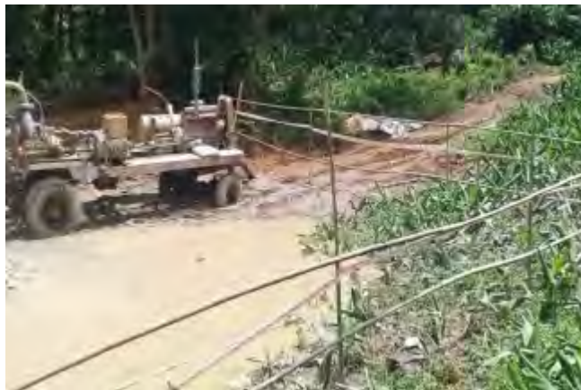
Bamboo barricading noted at work site
