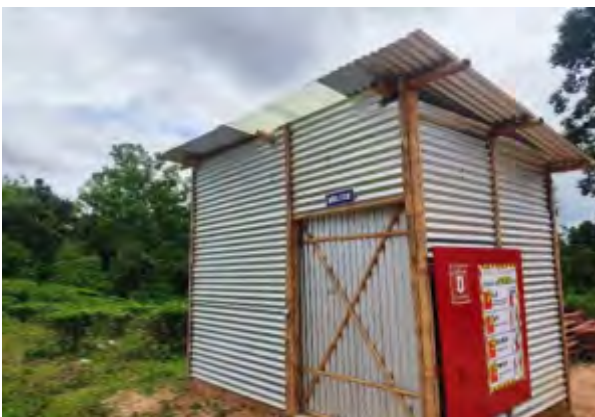
Diesel store at site
